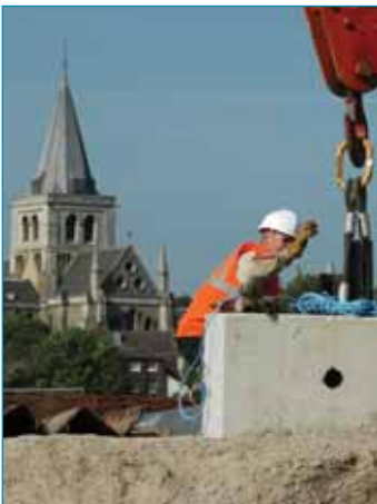
Rochester Riverside ready for development
