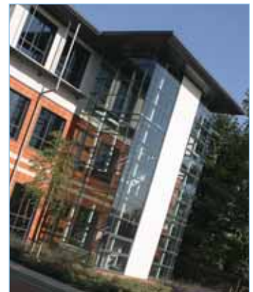
North Farm Industrial Estate, Royal Tunbridge Wells
