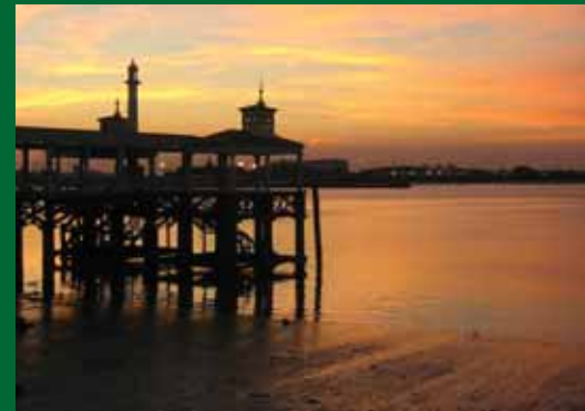
Gravesham's town pier
